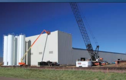
The Integra Plastics plant near Brandon.
