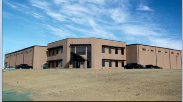
The Worthington Ag Parts building is nearly complete in Sioux Empire Development Park VII.
