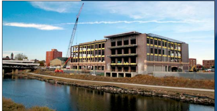
CNA Surety building under construction.
