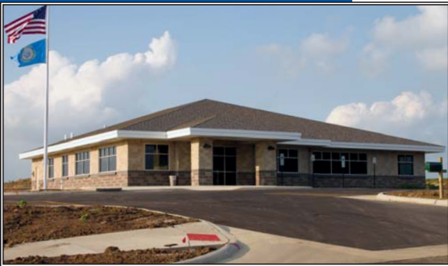
Recent construction projects in the Development Parks include the expansion of the Broin headquarters, above right; the completion of the Pulizzi Engineering facility in Park VII, above, and the Dakota Kitchen & Bath expansion, below right. The earthwork adjacent to Dakota Kitchen & Bath, seen in the foreground, is preparation for footings for the new Empire Plastics building in Park IV.
