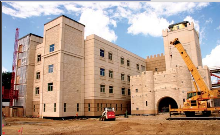
Work continues at Sanford Children's.
