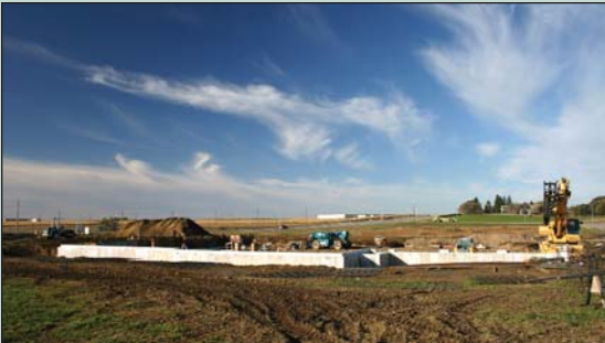
Construction has begun at the new Lions Eye Bank site.
